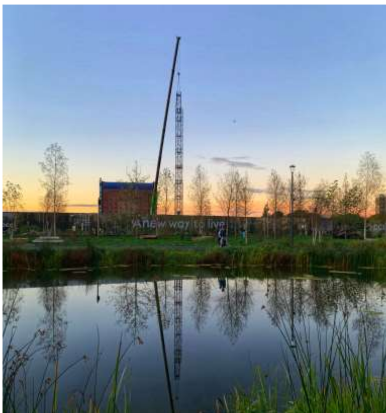
First tower crane being erected at Brent Cross Town
