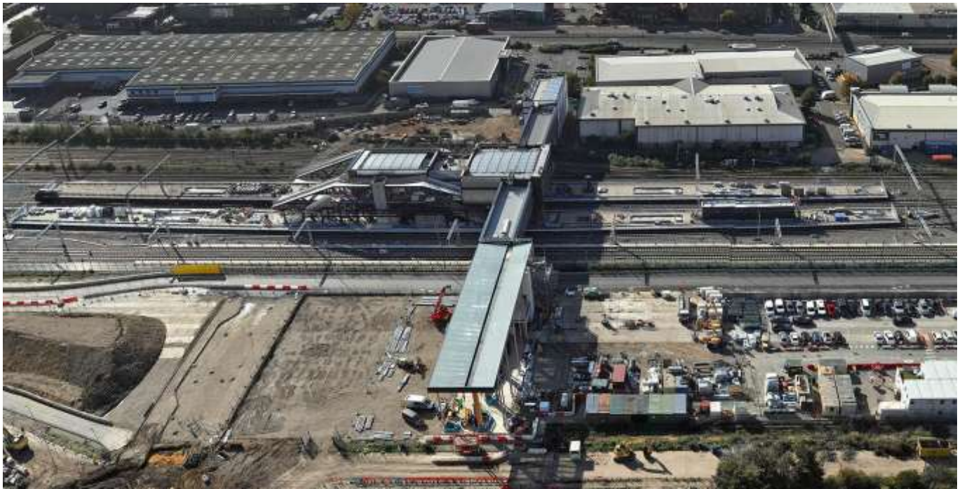
Figure 1 - Brent Cross West Station (October 2022)
