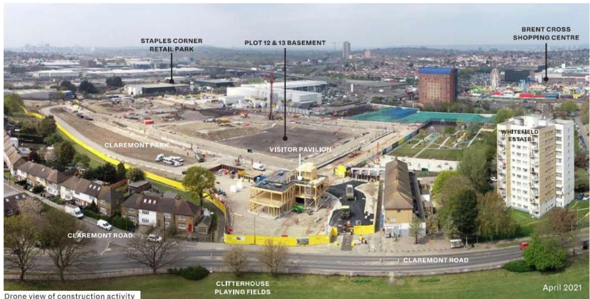
Brent Cross Town construction activity
