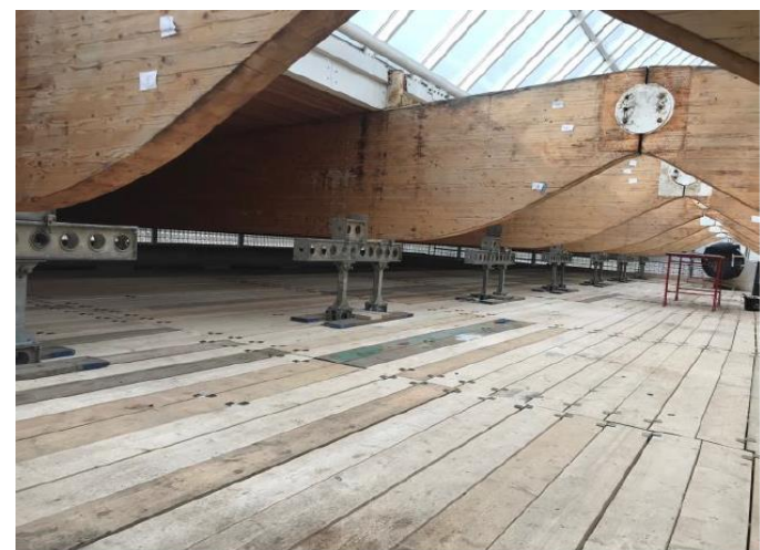
Structure: Access to timber beams and connections
