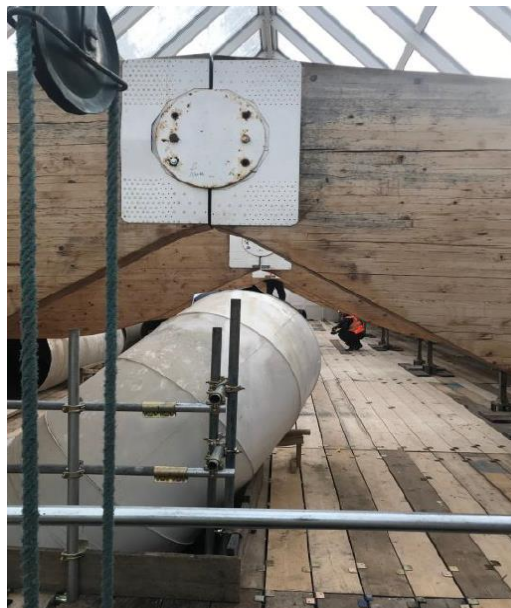
Access: Removal of ducting and apex connections
