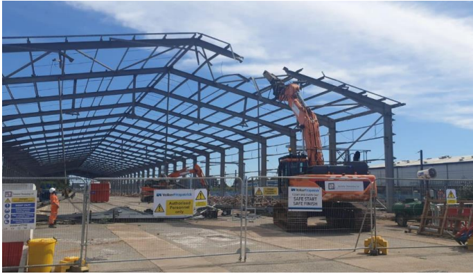
Jerich Shed Demolition
