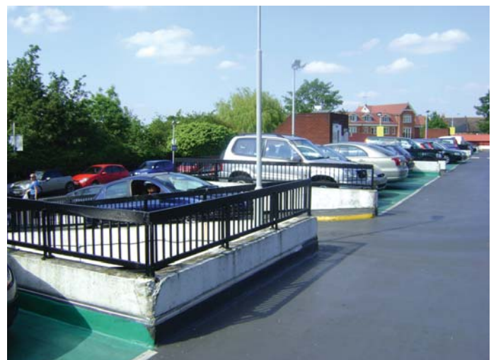
Tesco multi-storey car park
