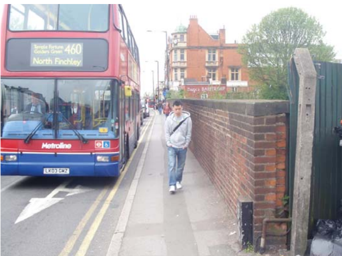
The bridge over the railway lines
